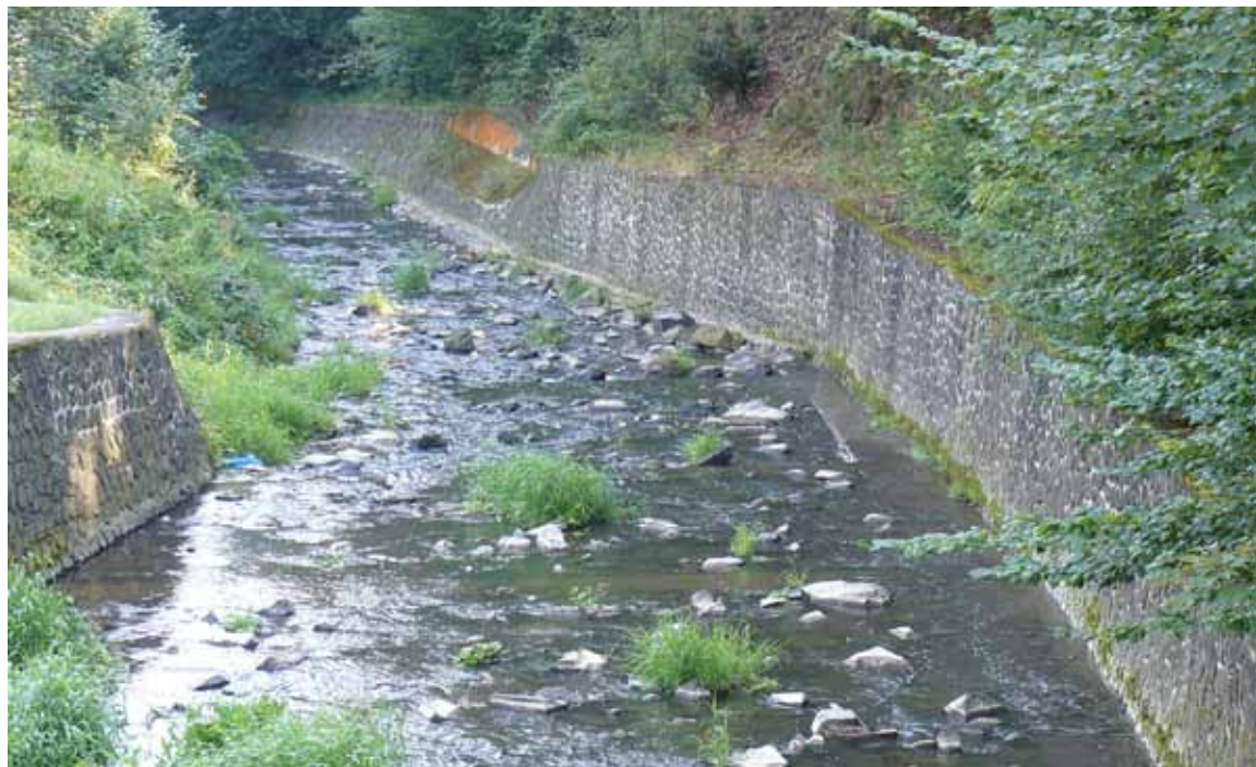
Fig. 3.7. Technical stream regulation that transforms a positive landscape element into a migration barrier.
