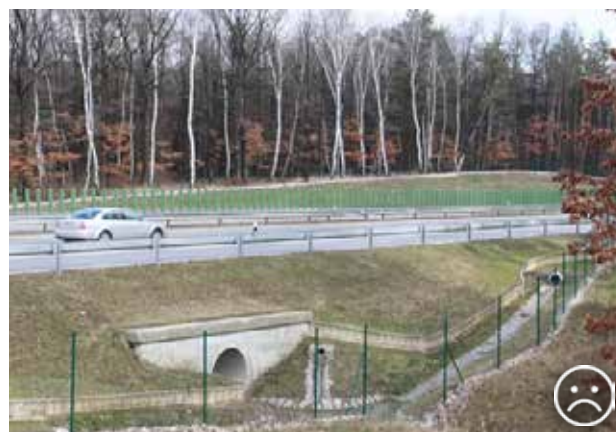
Fig. 10.45 If the entrance into a culvert is on one roadside outside of a fenced area and on the other roadside inside of the fenced area, animals using such an underpass stay trapped between the fences and the road. In case both entrances are inside a fenced area the underpass cannot be used by animals at all. © Václav Hlaváč
