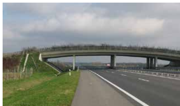
Fig. 6.42 A green bridge can be built even in a flat lowland area where the motorway is at ground level with the terrain. Connecting the bridge to the surrounding terrain however represents a more extensive land occupation compared to a situation where the motorway leads in a notch. Motorway M7, Hungary. © Ábrahám László
