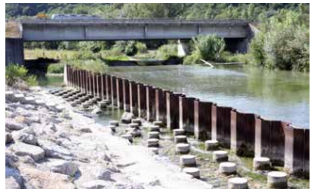
Fig. 10.50 A fish crossing near Lyon, France, where a vertical step on a watercourse was created as a result of a road construction. The fish crossing is placed directly in the watercourse and is used by the entire fish spectrum inhabiting the stream. It is also used by otters. © Václav Hlaváč
