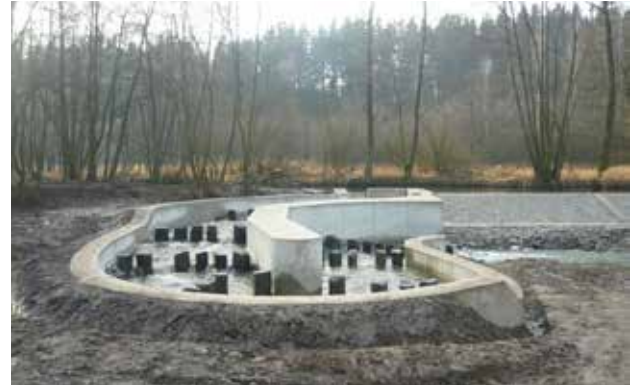
Fig. 10.49 A fish crossing in the form of a bypass – in order to overcome a weir 1.3 m high, it was necessary to create a fish crossing with a total length of 40 m. The Czech Republic. © Bohumila Jermlová
