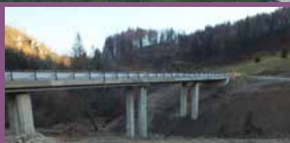
B) Building of a new bridge on pillars – the corridor is partially functional. It is necessary to plant guiding vegetation under the bridge and in its surroundings. © Drahoš Blanár
