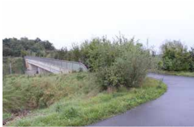
Fig. 10.17 A forest path over a motorway widened by stripes of bushes on both sides allows for the connection of forest environment for many species including mammals living on trees, small birds or bats. It represents a very affordable measure with a strong effect. Dresden, Germany. © Václav Hlaváč
