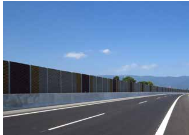
Fig. 4.8 A noise protection wall eliminates the effect of disturbance while also increasing the barrier effect. © Tomáš Flajs
