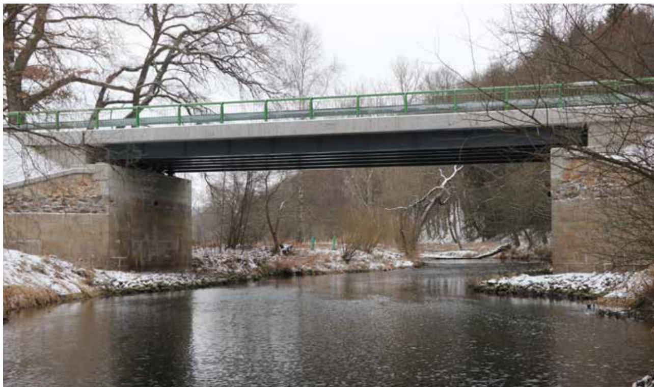
Fig. 10.1 Bridges over watercourses can easily be adjusted in a way that allows animals to use them to safely overcome a road. It is necessary to keep natural banks that fluently continue in the surrounding terrain. © Václav Hlaváč
