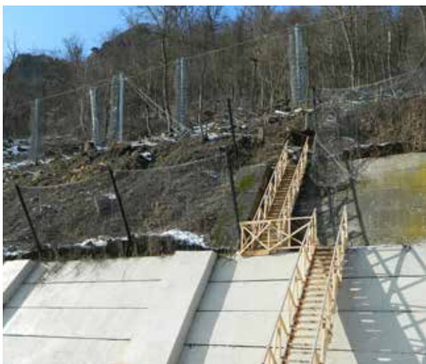
Fig. 9.13 Steep slope secured by a catch fence or wire mesh against falling stones. These measures are sometimes necessary to stabilize slopes, but at the same time they represent a reinforcement of the barrier effect and the destruction of road verges as natural habitats. If possible, a more gentle solution should be preferred. R2, Zvolen, Slovakia. © Miroslav Jarný
