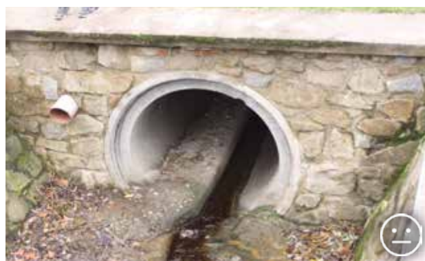
Fig. 10.44 Usability of culverts for animals can be increased by creating a dry concrete bank which allows for the movement of terrestrial animals. © Václav Hlaváč
