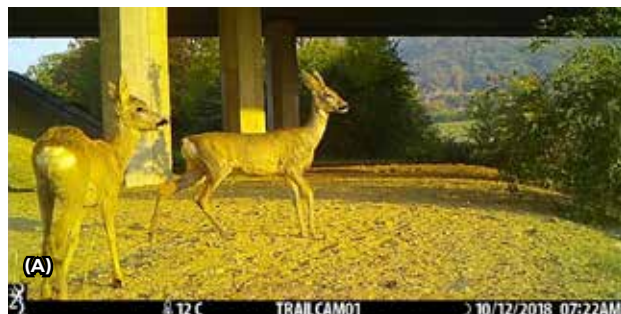
Fig. 10.36 Special underpasses for large mammals are built in places where a motorway crosses a migration corridor. D1 motorway, Bělá, Czech Republic © Martin Strnad
