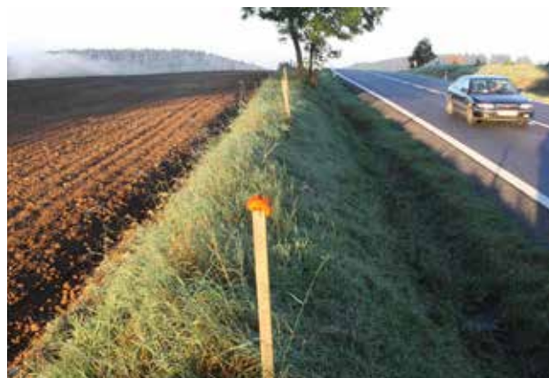
Fig. 10.59 Olfactory deterrents are used in many areas of the Czech Republic. Their purpose is to alert ungulates (especially the roe deer and the wild boar) that they are in a dangerous area. However, these deterrents only seem to have a short-term effect; real decrease in the number of accidents with fauna due to this method has not been proven yet. © Václav Hlaváč
