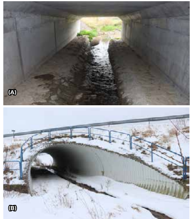
Fig. 10.42 Different types of bridges over small watercourses are very well usable as fauna passages for small animals. Dry banks at least 0.5 m wide allow the movement of a broad spectrum of species up to the size of badger. The banks should be made from stone pavement and concrete should be avoided, because it does not allow migration of amphibians (risk of drying out). © Václav Hlaváč
