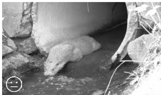
Fig. 6.35 Culverts can – with a suitable design – serve as fauna passages for many animals. Rectangular shape is always the preferred solution. Tube culverts are not an optimal solution, but otters are able to use them at times of lower flow rates. © Václav Hlaváč, phototrap picture
